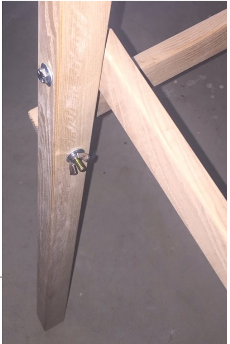
Figure 10: Left upright pair with horizontal brace (back) and diagonal brace held by 2" hex bolt
