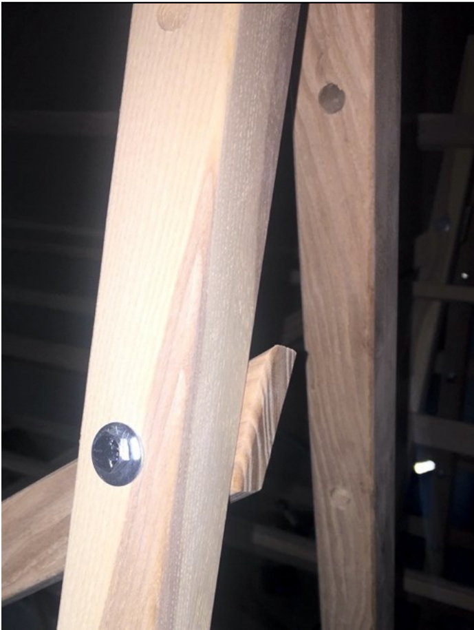
Figure 11 Diagonal brace from the lower left (bottom of left upright) to the upper right (top of right upright)
