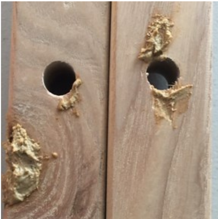
Figure 3. Filler surrounds defects in drilled holes and a knot in a pair of upright boards
