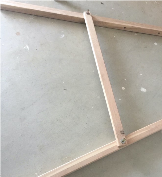
Figure 9: Horizontal cross brace near bottom of upright pair using 3" hex bolt and wing nut. (Note: both uprights have a brace, located on the outside of the uprights as they are being faced)
