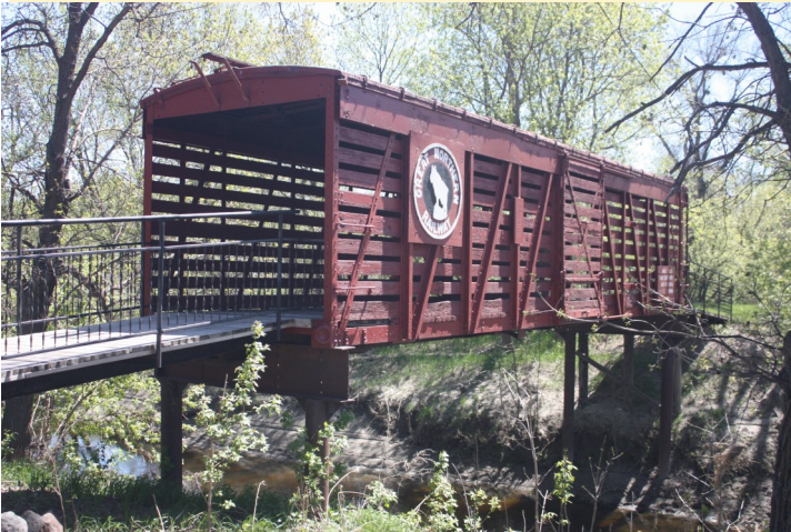
Arglye, MN: Turn an old, unused freight car into a bridge for access within a park.
