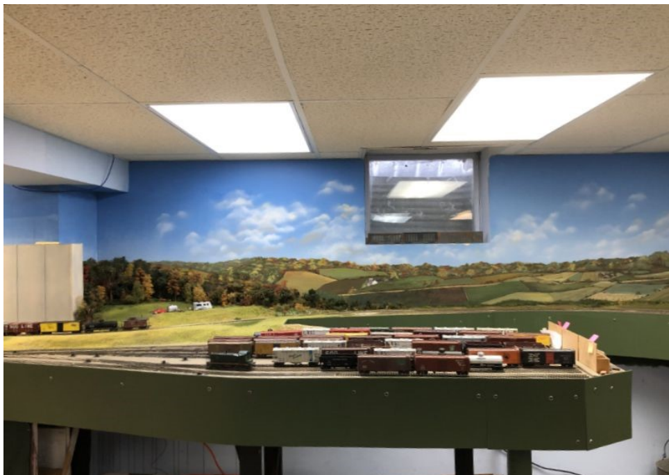
The finished fixture is brighter, and has more even lighting than the old tubes.
