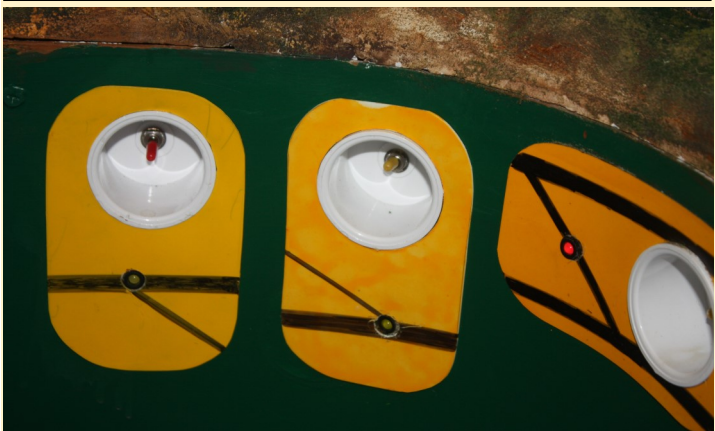
Joe Robertson, MMR Kansas City, 2018: Recess the toggle switches for turnout control to prevent accidental route changes. With a bi-colour LED, show the route alignment.
