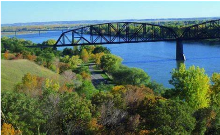
View of the Northern Pacific Railroad bridge crossing the Missouri
