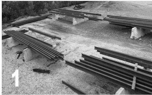
Photo 1 shows Rail stored off the ground.
